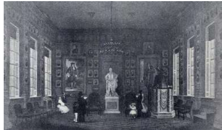
INTERIOR OF INDEPENDENCE HALL.
